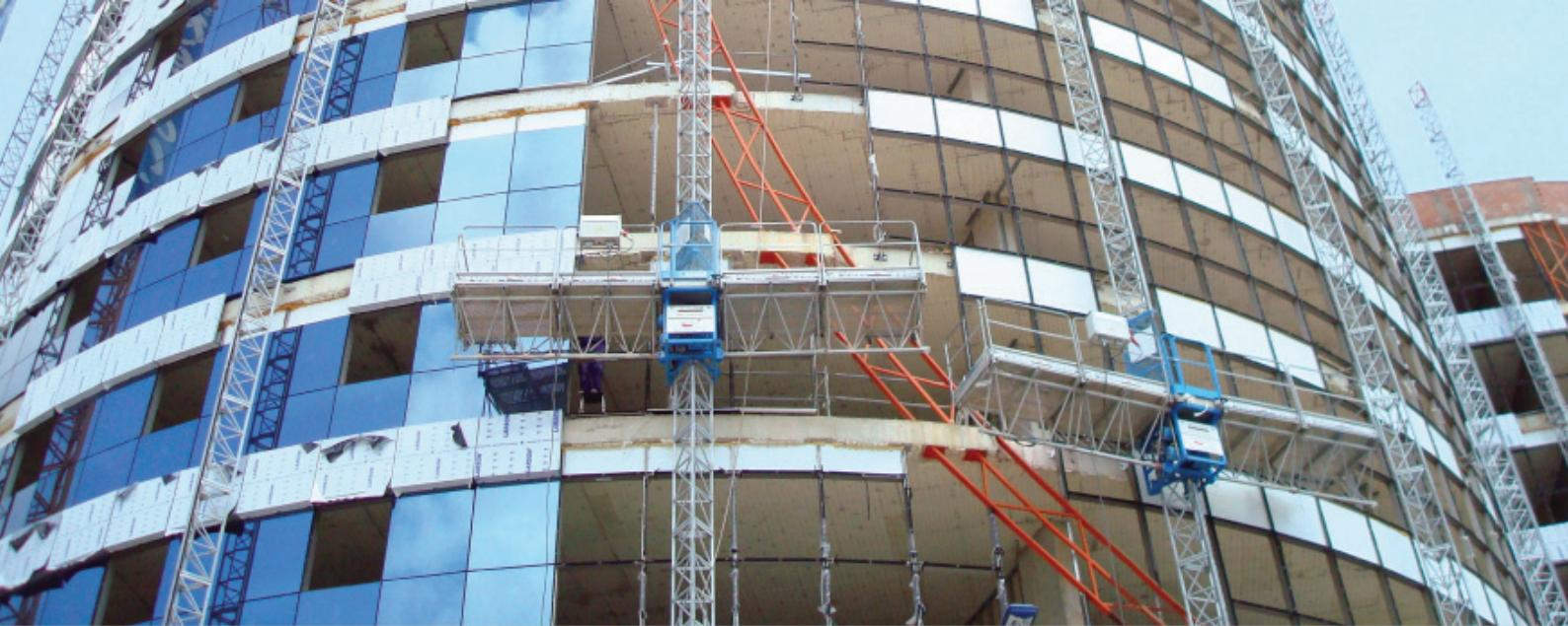
Within the Azor Group, **Eletor 2000** is equipped with over 1000 electric motors on mast-climbing work-platforms to enable work be carried out on any facade.
